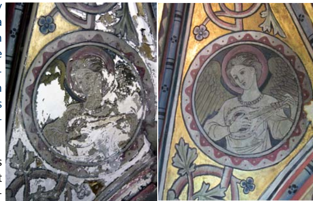
Ceiling panel with roundel before (left) and after (right) treatment.
