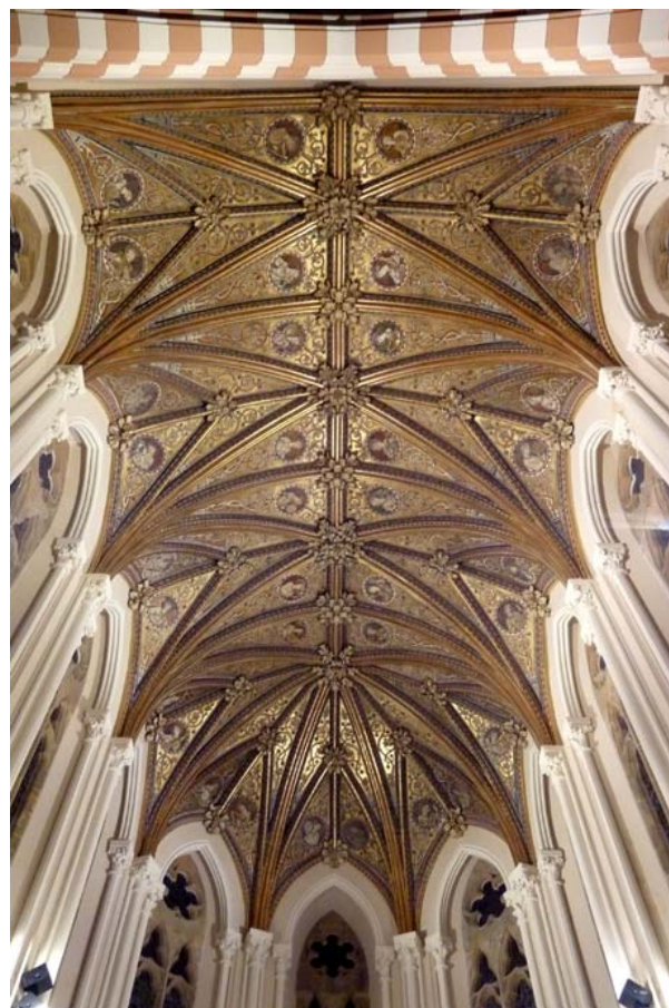
Chancel ceiling after conservation and restoration.
