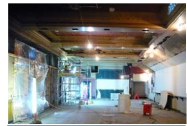
Plaza Cafe during renovation, 2009.
