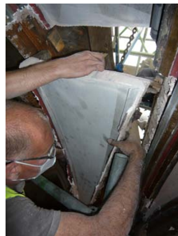
Panel being carefully removed.
