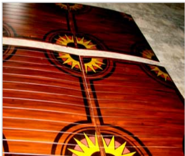
The new stencilled panels created to cover the plastered 'balcony' section of the ceiling.
