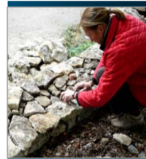
Rebuilding of the dry stone wall
