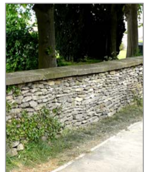
The reconstructed dry stone wall retaining its original materials
